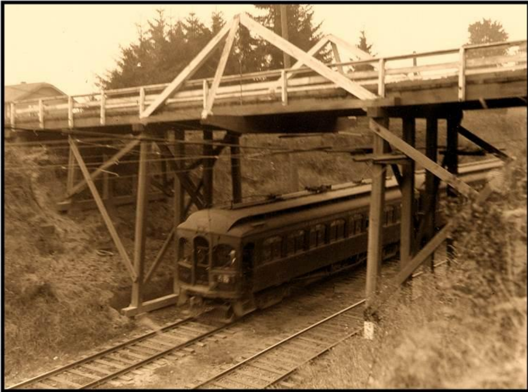
An Oregon Electric train passes under an overpass at 19th near Multnomah.
